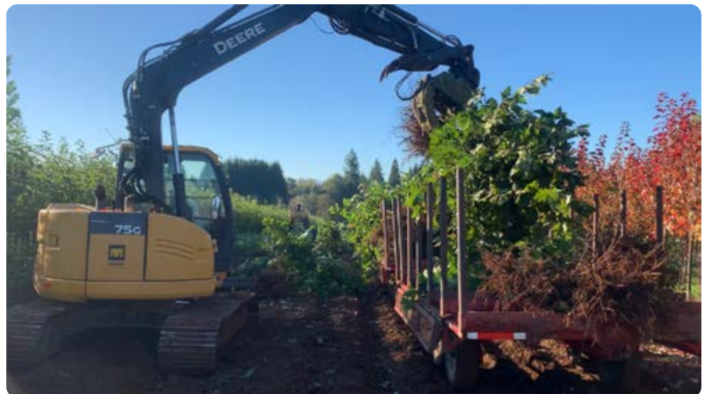
Marco Francisco operating the excavator and loading bulking trailers with the grapple.
