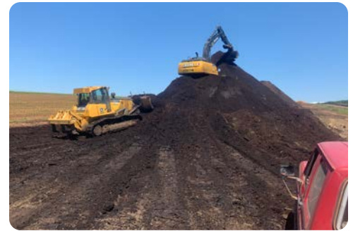
Luis DeLucio in the dozer and Jeremy Imes in the excavator work together to pile 7,000 yards worth of compost!
