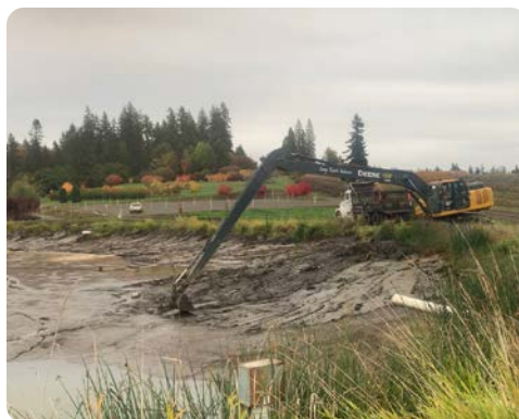
Jeremy Imes in the long reach excavator and Jorge Magaña in the dump truck team up to rid the Cottrell pond of mud.
