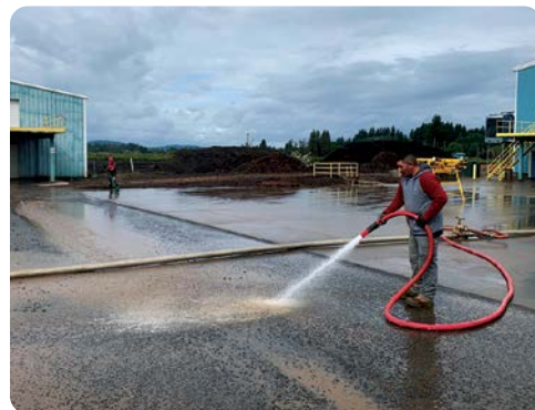
Ricardo Vázquez (foreground) and Welfri Sales wash the mud, nails, and rocks off the concrete in front of cooler #7.
