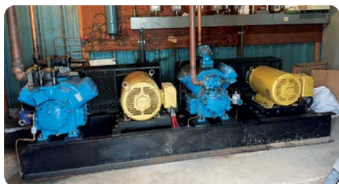
Compressors and accumulators do their work in the mechanical room in Hood Acres cooler #5.
