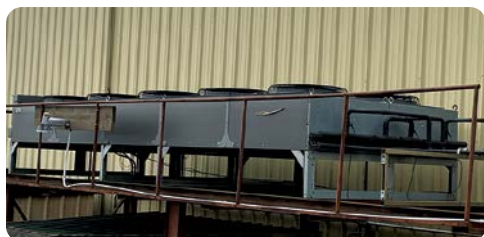
At the Barlow cooler, fans on the outdoor condenser unit take the heat removed from inside the building and release it to the open air outdoors.
