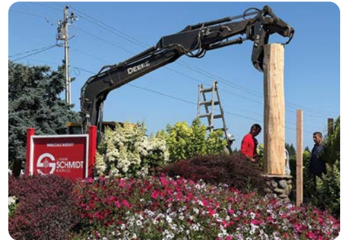
Gordy Webster and the maintenance crew setting posts for the newly refurbished main entrance sign.
