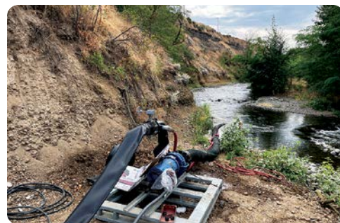
New pump and suction line set up and ready to go
