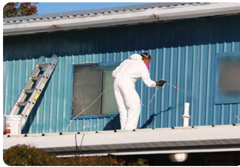
Travis Baie paints the upper story of the main office.
