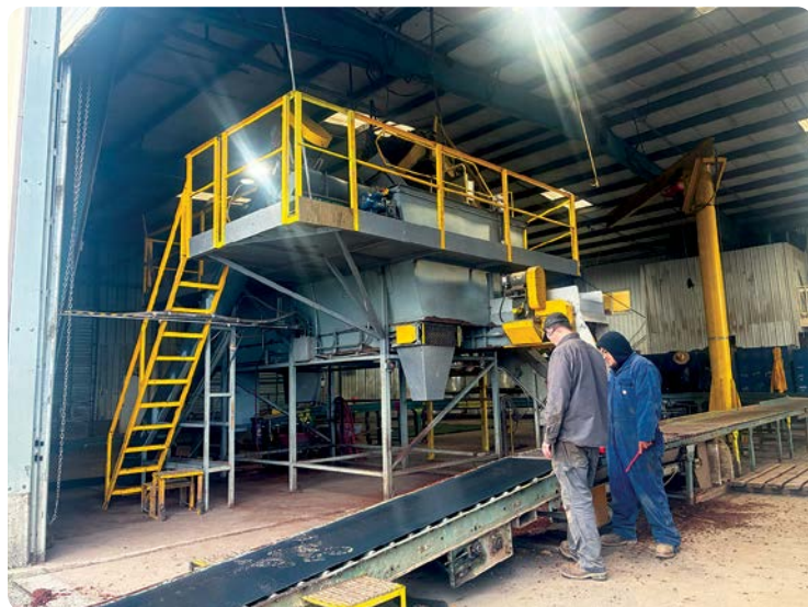
Zac Hall and Isauro Francisco Jr. inspect their belt replacement on the CF north potting line.
