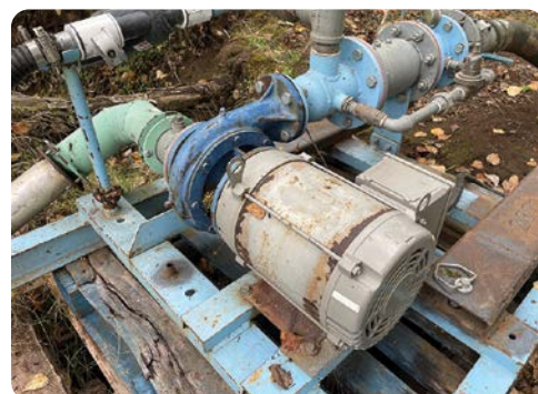
Example of a centrifugal style water pump. Generally used to pump water from a pond or river.
