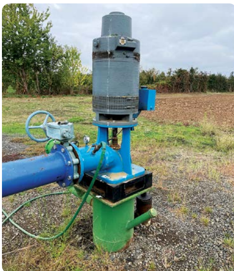
Example of a turbine style well pump. Electric motor on the surface, pump down the hole
