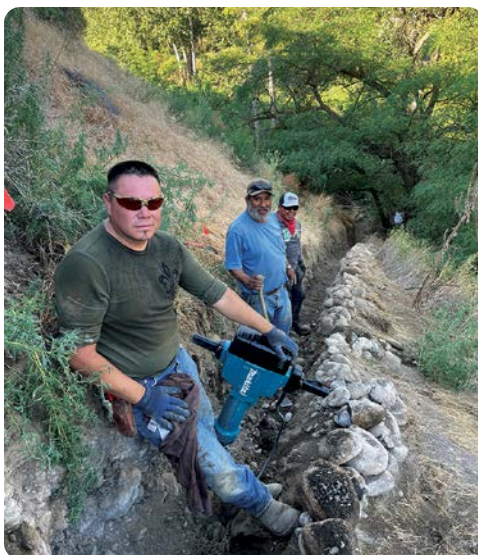
Abraham Ibarra, Aurelio Gonzales, and Rogelio Hernandez work with jack hammers, pick axes, shovels and hand moving of big stones to trench a 30% slope for the new irrigation main line. This was hard work!
