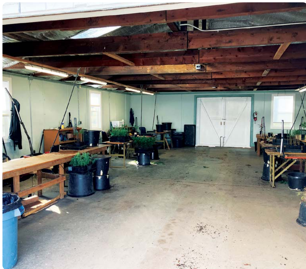
New windows and skylights add much needed light to the new grafting house.
