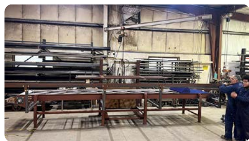
Mudzilla in the early stages of construction at the Hood Acres fabrication shop.
