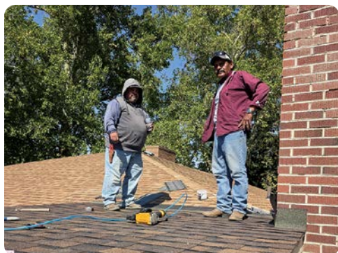
Miguel Reyes and Oscar Ponce making roof repairs to a house on our farm making sure its winter ready.
