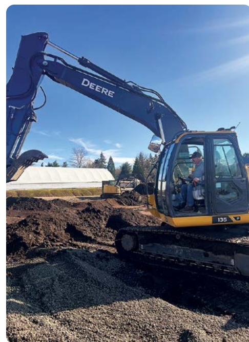
Jeremy Imes operating the large excavator, with another excavator and the dump truck in the background to clear the way for our new gravel yard.
